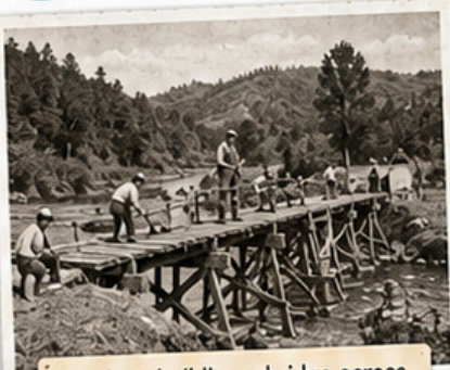
Workers building a bridge across the Wharekawa River, 1952.
